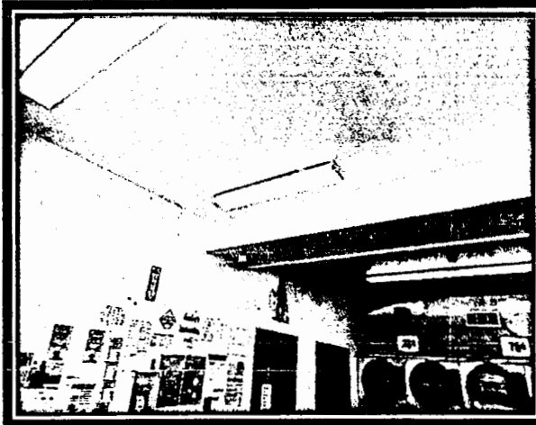
Photo 31: Inside of Laundry Mat
