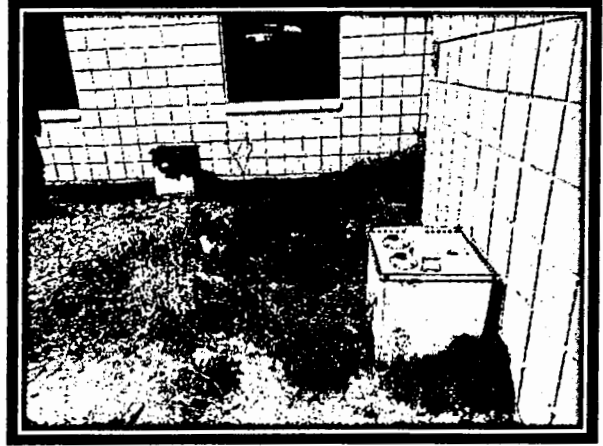
Photo 14: Hospital Grease Traps with Release
