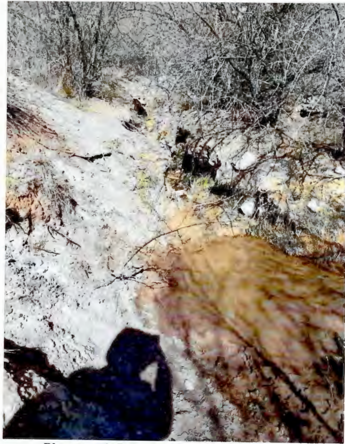
Photograph 7: Seep within Riparian Habitat
