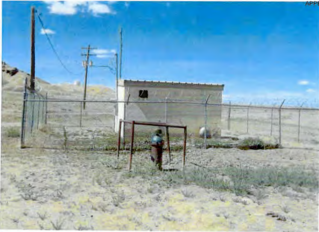
Looking Northwest at NTUA water well & tank in Section 9 (25n-19w)
