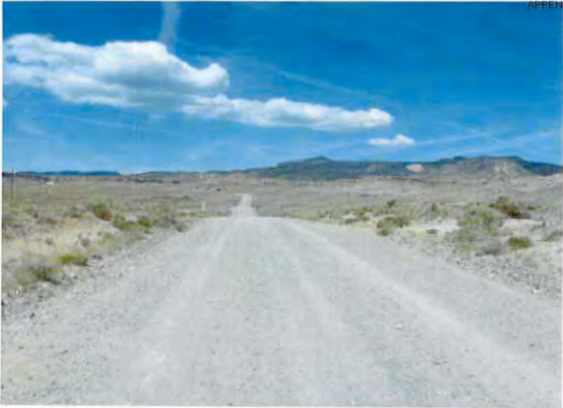
Looking West at gravel N-5016 in Section 28 (26n-19w)
