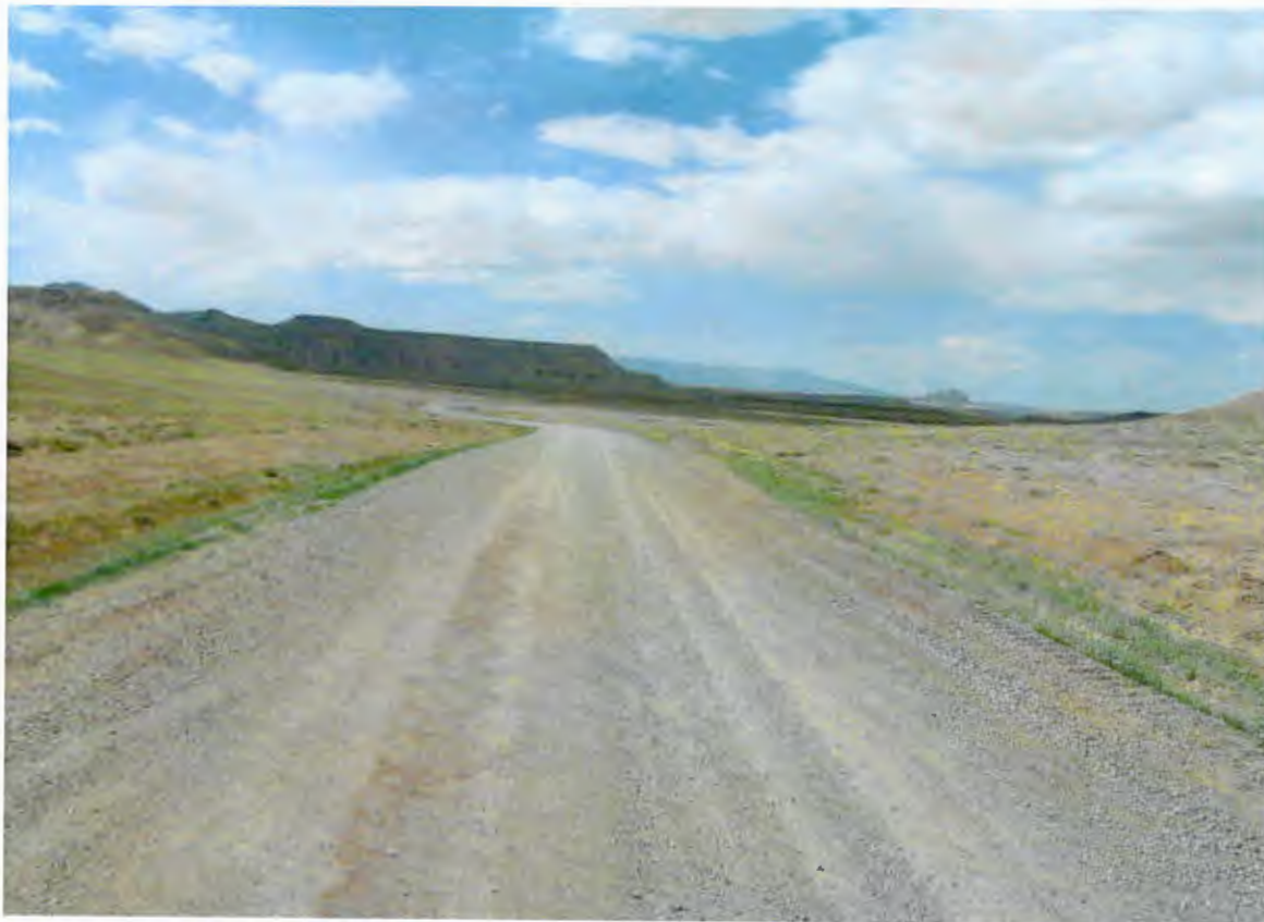
Looking Northwest at N-5012 in Section 17
