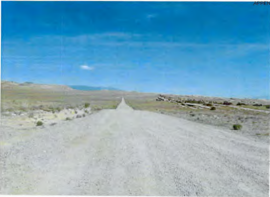
Looking North at gravel N-5012 in Section 21 (26n-19w)
